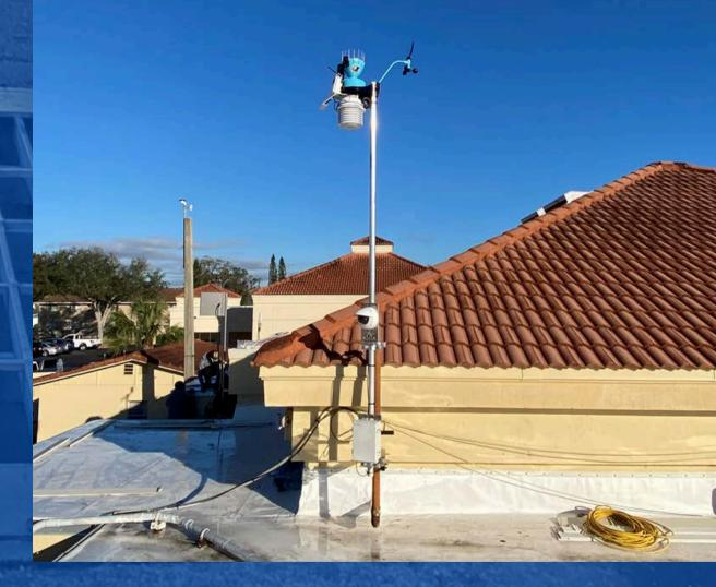
The City has installed a weather station atop City Hall that measures atmospheric conditions which will be used to document our stormwater system's performance compared to measured rain events.
